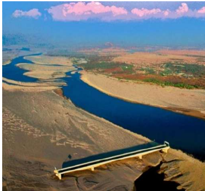
Image 1 - Choluteca Bridge in Honduras
